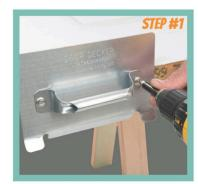
ATTACH A DOOR DECKER BRACKET TO THE APPROXIMATE CENTER OF EACH END OF A DOOR USING THE ENCLOSED OR SIMILAR SCREWS, MAKE SURE THE DOOR DECKERS ARE INSTALLED IN THE SAME DIRECTION, (HOLLOW METAL DOORS REQUIRE SELF TAPPING SCREWS WHICH ARE NOT INCLUDED WITH YOUR PURCHASE,)
